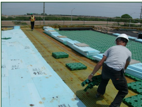
Installation of plastic trays
