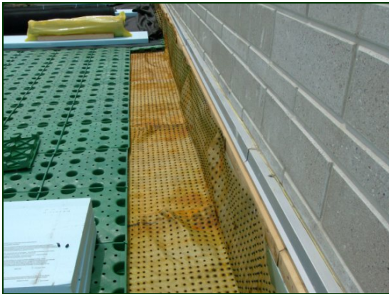
Installation of Biobarrier on parapet wall
